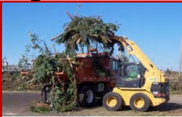
A. Debris Clearance
